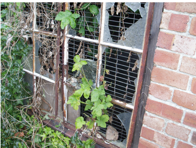
Damaged windows and failing frames, west elevation
