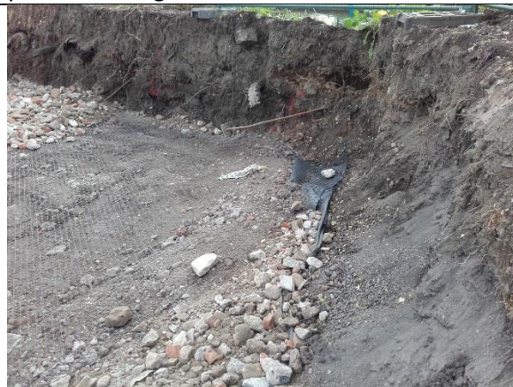
Pile mat 3 excavation – granular Made Ground
