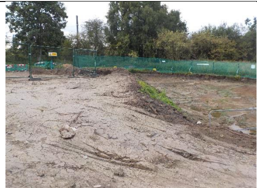
West GUC pile mat excavation in lower eastern fill section
