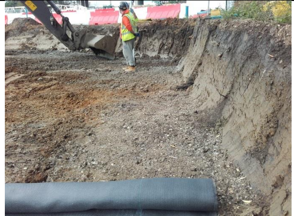
Pile mat 2 (river east platform) – formation level
