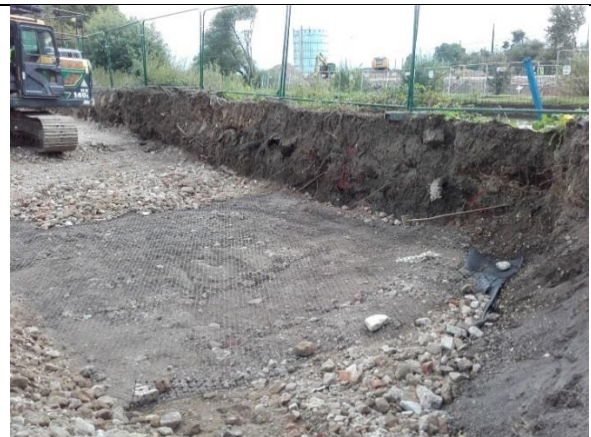
Pile mat 3 – placement of Class 6F2 on geotextile and lotrak geogrid
