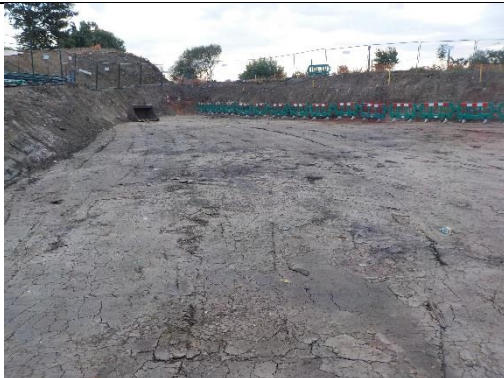
West GUC pile mat excavation completed in upper western section
