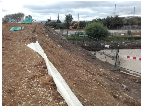
Lagoon bund crest – no signs of major instability
