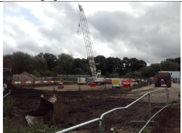
Pile mat 1 complete.
