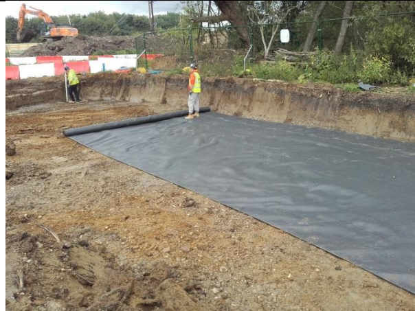
Pile mat 2 (river east platform) excavation and placement of geotextile
