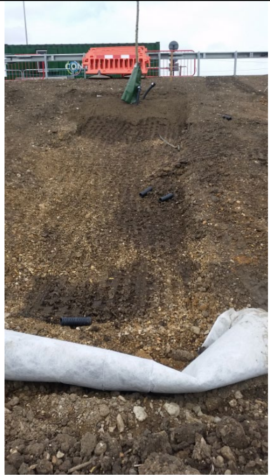
Photo 6 Completed installation and backfilling of tree pits.
