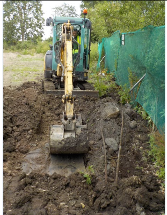
Photo 6 Railway triangle slit trenches exposing hardcore and geotextile placed to form hardstanding during construction works.
