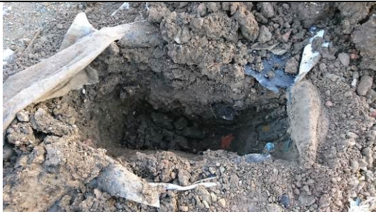
TP2 excavation to 1.0m bgl
