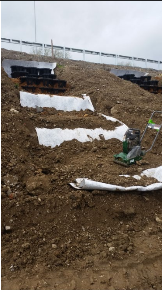
Photo 5 Compacting fill on geotextile and benching following tree pit installation.
