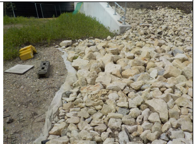
Photo 4 Completed rock scour protection on Terram geotextile separator
