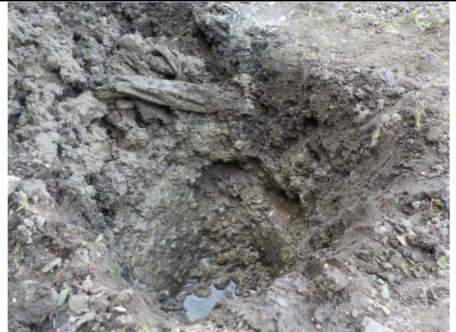
Photo 2 Unsuitable 'Topsoil' stockpiled in lagoon – removed off site for disposal.
