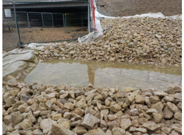
Photo 2 East YB south scour protection. Larger stone to be placed at slope toe.
