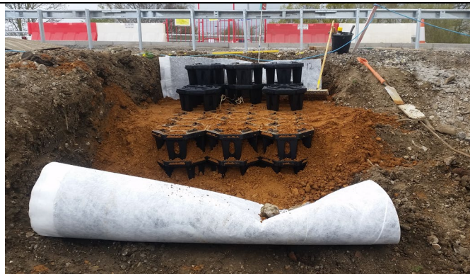
Photo 3 Tree pit installation in Zone 4.
