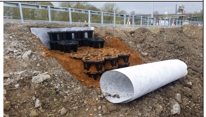
Photo 4 Tree pit installation in Zone 4.
