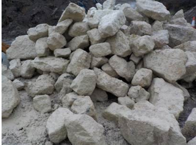
Photo 1. Scour Protection – imported large stone (prior to breaking)
