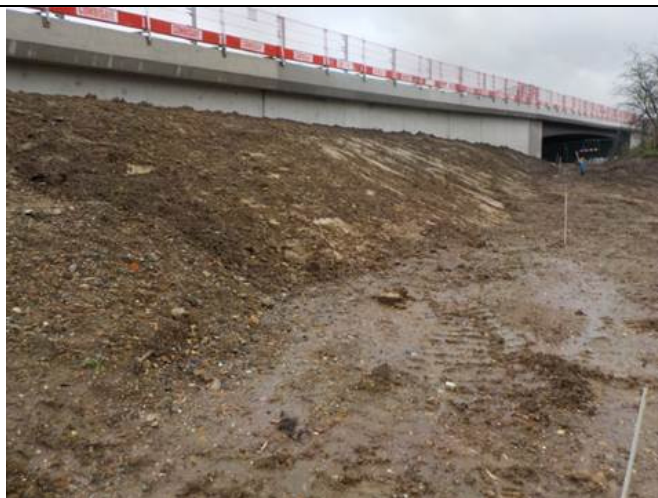
Photo 5 Newly placed landscape fill to West GUC south wing wall
