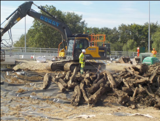
Photo 1. Jet washing timber from stockpile SP2 to remove invasive species spores prior to disposal off site.
