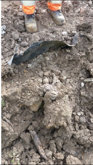
Photo 1. Example of material sampled beneath liner in lagoon.
