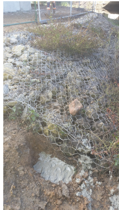
BH3 decommissioned and grouted
