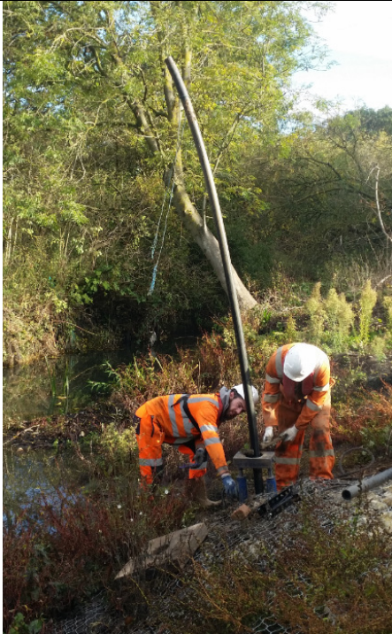
Decommissioning of Bh3 adjacent to Yeading Brook
