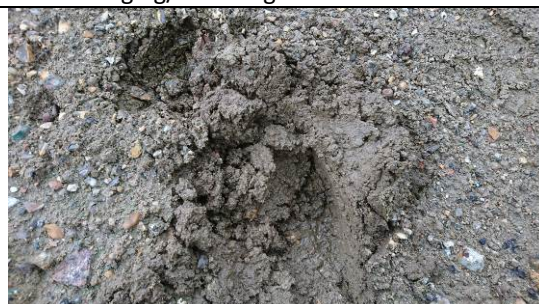
Fines slurry saturated with ponding surface water
