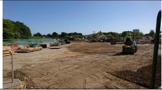
Fill works to Pump Lane area
