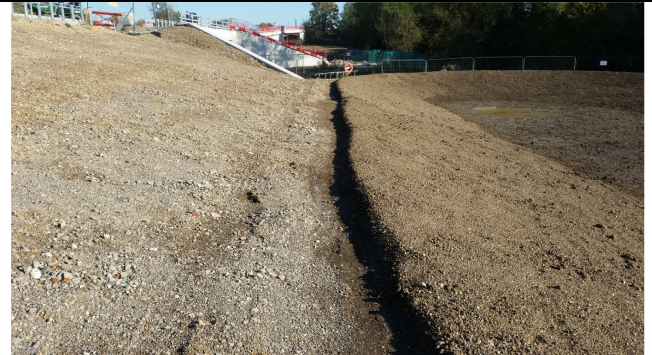
Top of Detention Basin along toe of Western embankment south.
