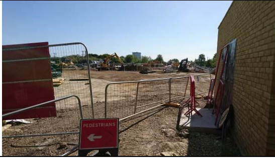
Fill works to Pump Lane area
