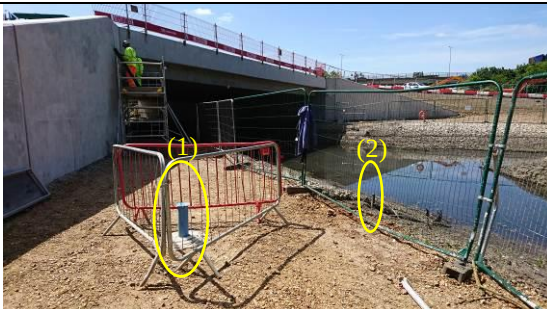
Replacement Environ borehole (1) and exposed open redundant borehole in Yeading Brook channel (2)
