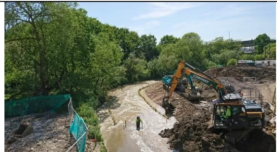
Bank widening, dredging and reed bed installation works along Yeading Brook
