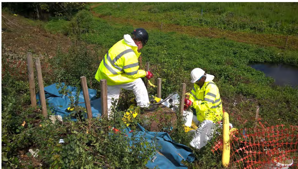
Photo 3. Decanting of liquid contents from damaged 205l drums to new plastic 25l containers for transport.
