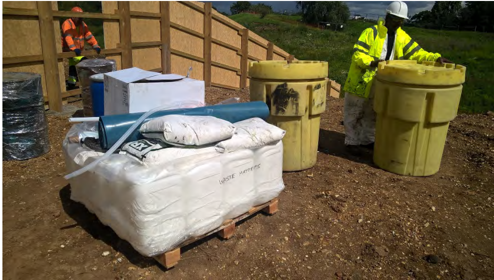
Photo 5. Preparation of waste containers for removal from site including placement of damaged 205l steel drums into over drums and palletising of 25l product containers.
