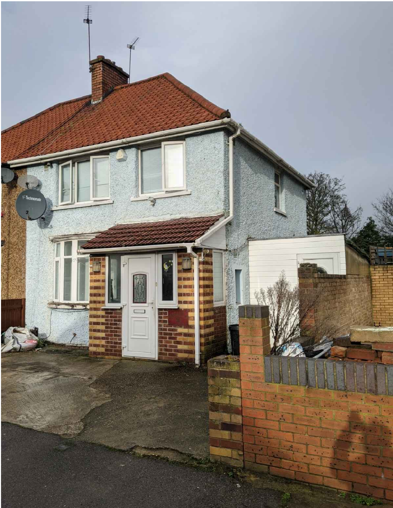
01 Site Photo - Main house (Street view)
