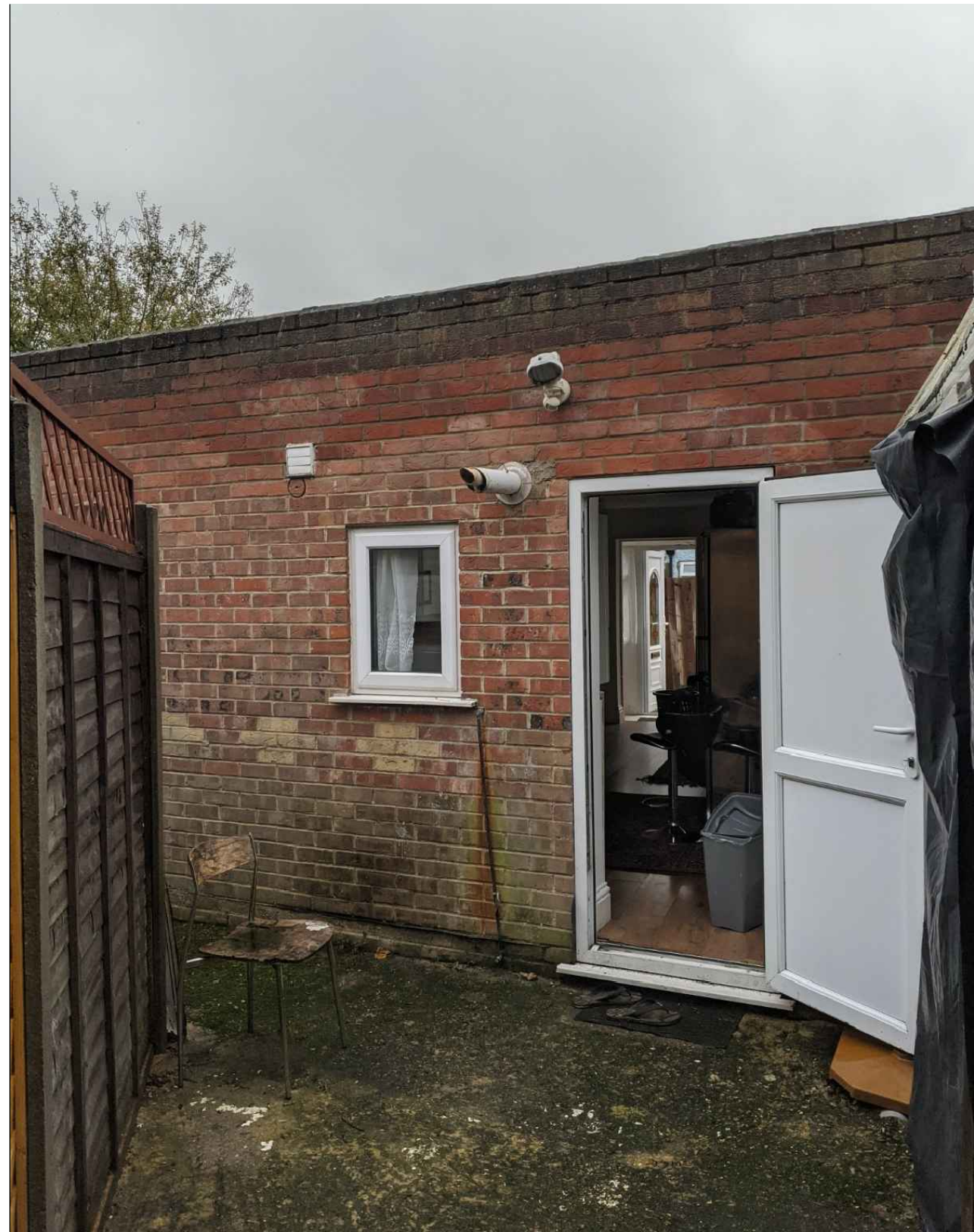
04 Site Photo - Rear outbuilding (Rear view)
