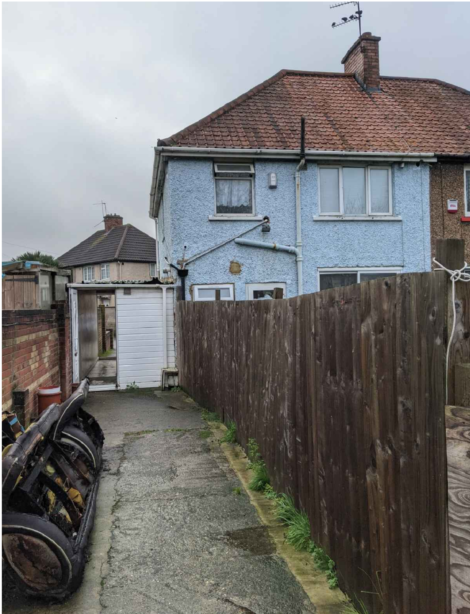
02 Site Photo - Main house (Rear view)
