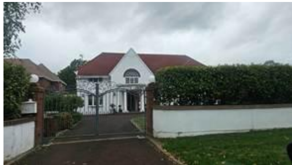
Traditional red-brick dwelling with roof accommodation and dormers.
