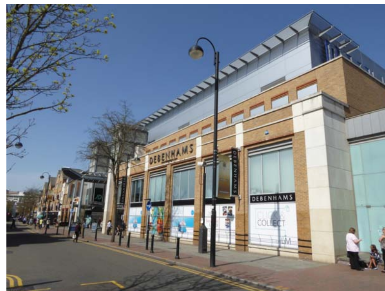
Existing facade - Looking North West from High Street
