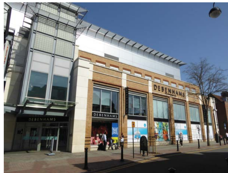
Existing facade - Looking North East from High Street
