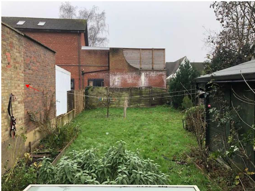
Fig 7, View to rear boundary. Note residential garage space to rear to which there is no impact. Timber shed to right of picture to be removed. Note, arrow marks extent of proposed development
