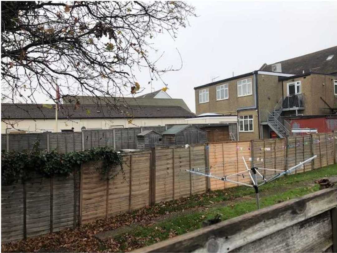
Fig 5, Additional side view to neighbours. Note single story extension
