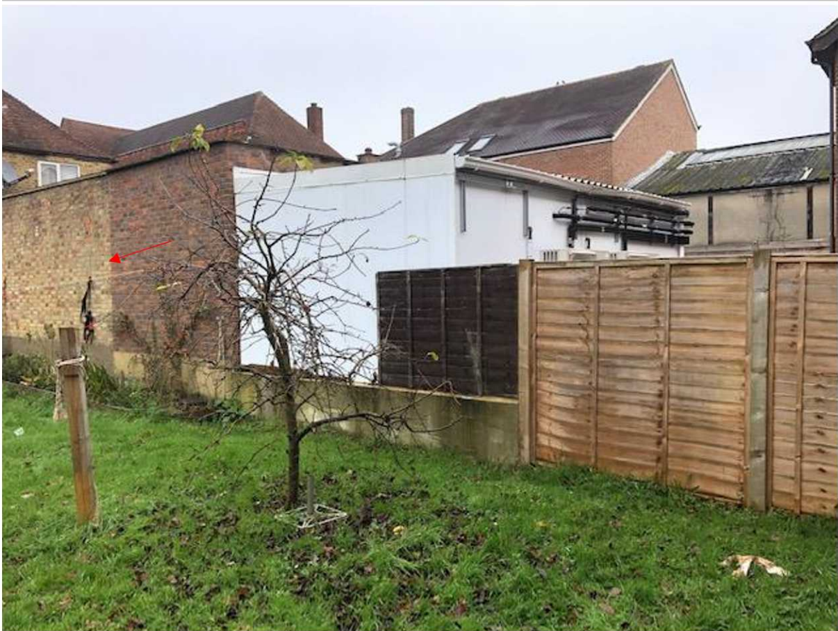
Fig 4, Side view from rear of development boundary. Note proposed development will not extend beyond the yellow brick, this leaves space from the red brindle brick and later Upvc refrigeration unit.
