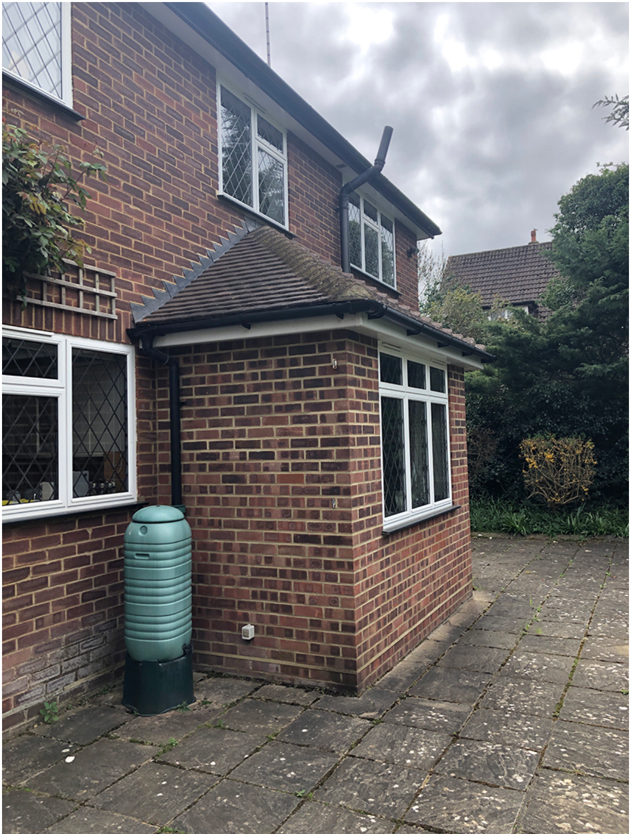
Side view looking toward boundary with No.29 Eastbury Road.
