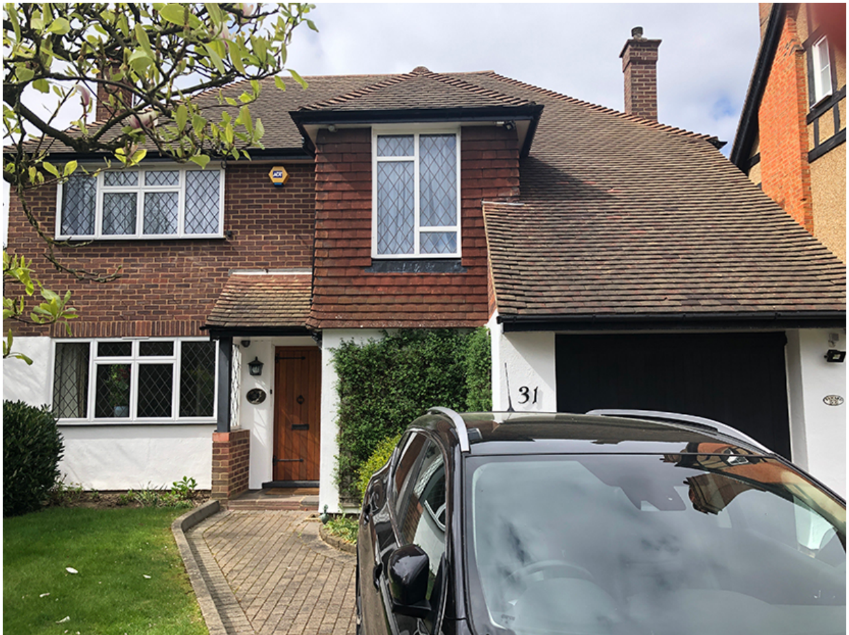
Front view from Driveway off Eastbury Road
