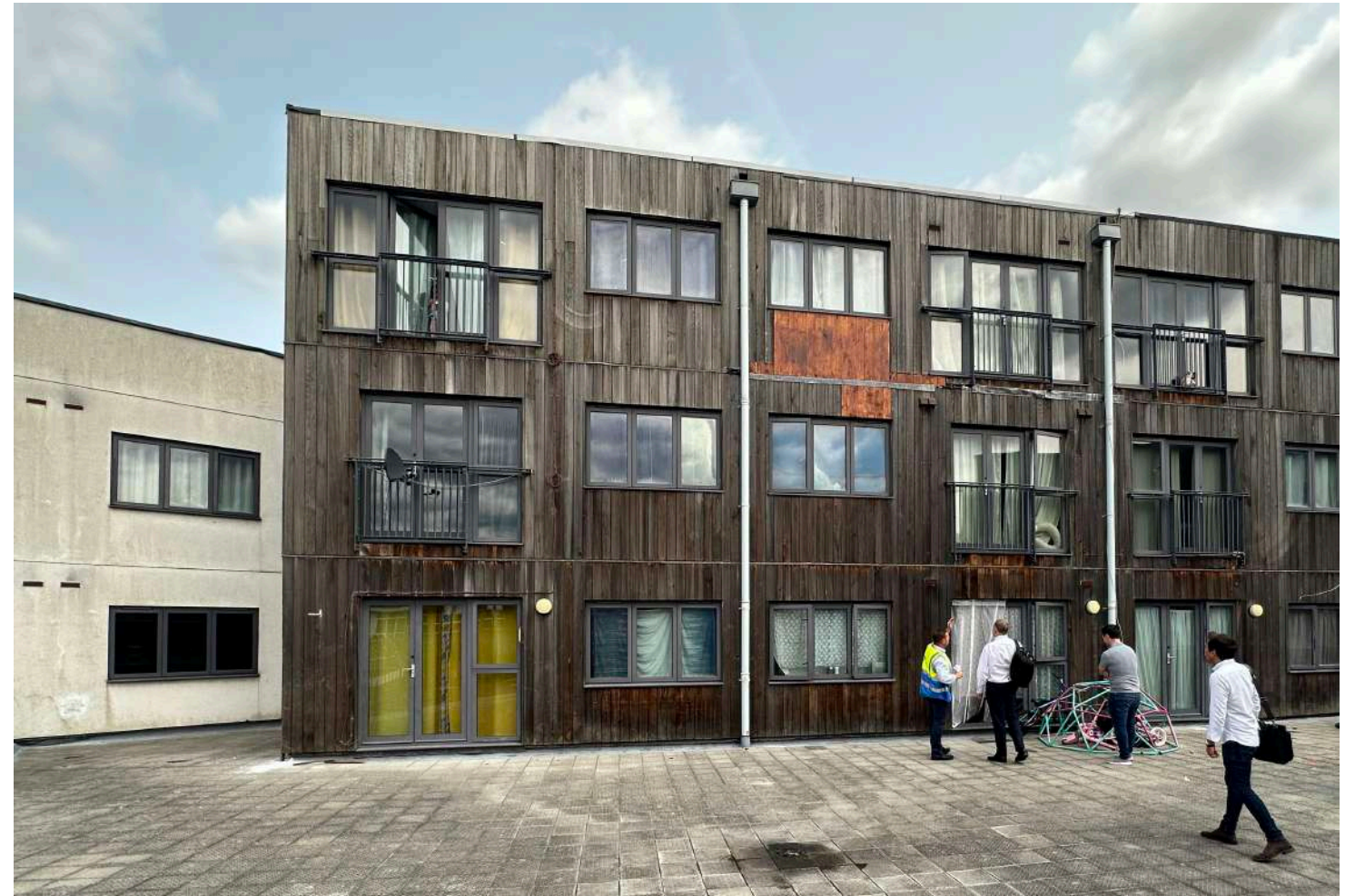
The rear of the building shows bad maintenance and patchy repairs that have been undertaken over the years.
