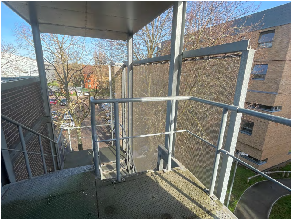
Existing guard rail on the third floor, proposed for removal
