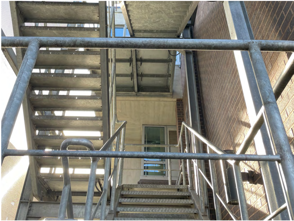
Guard rail detail from the first landing of the escape stairs
