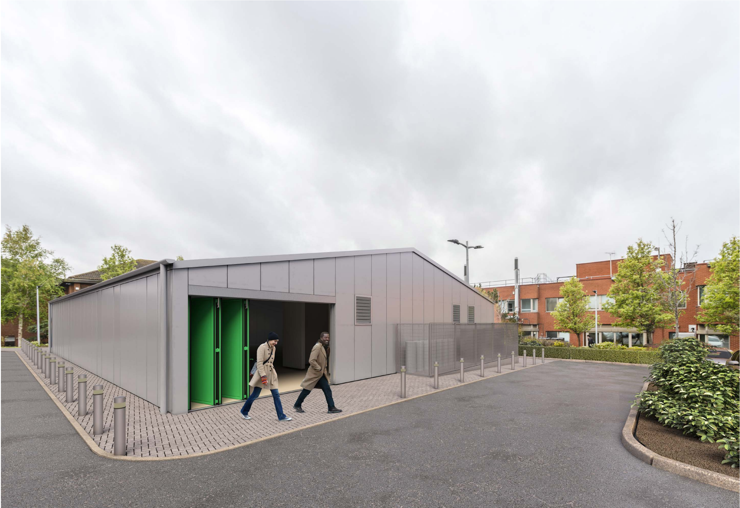
View of north east corner of building from the car park
