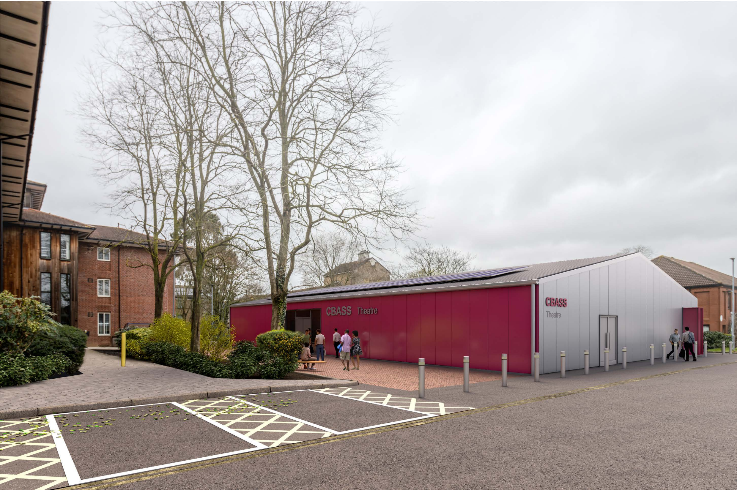
View of south west corner of Building 2 from West Spur Road
