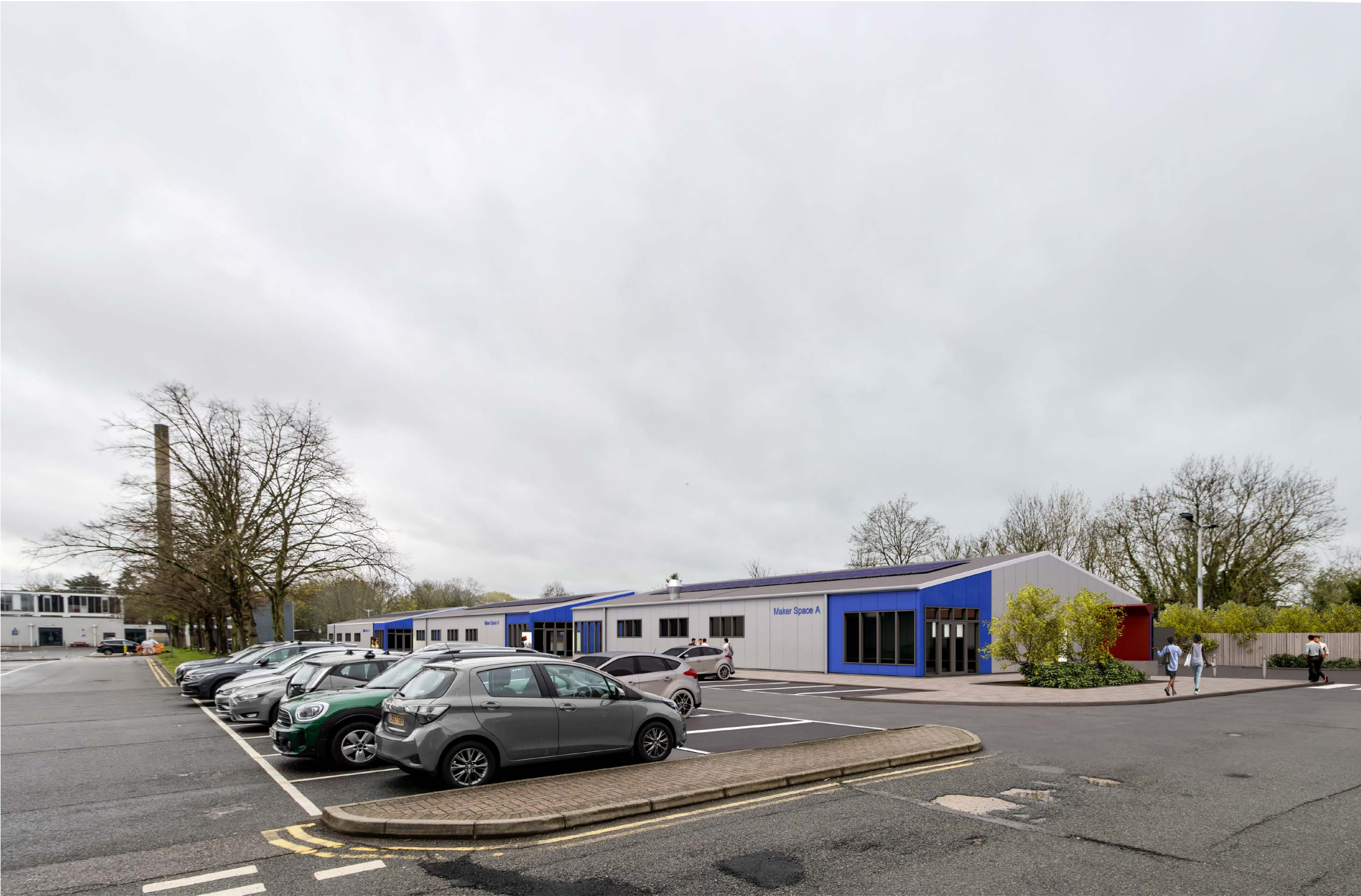
View of north east corner of Building 1
