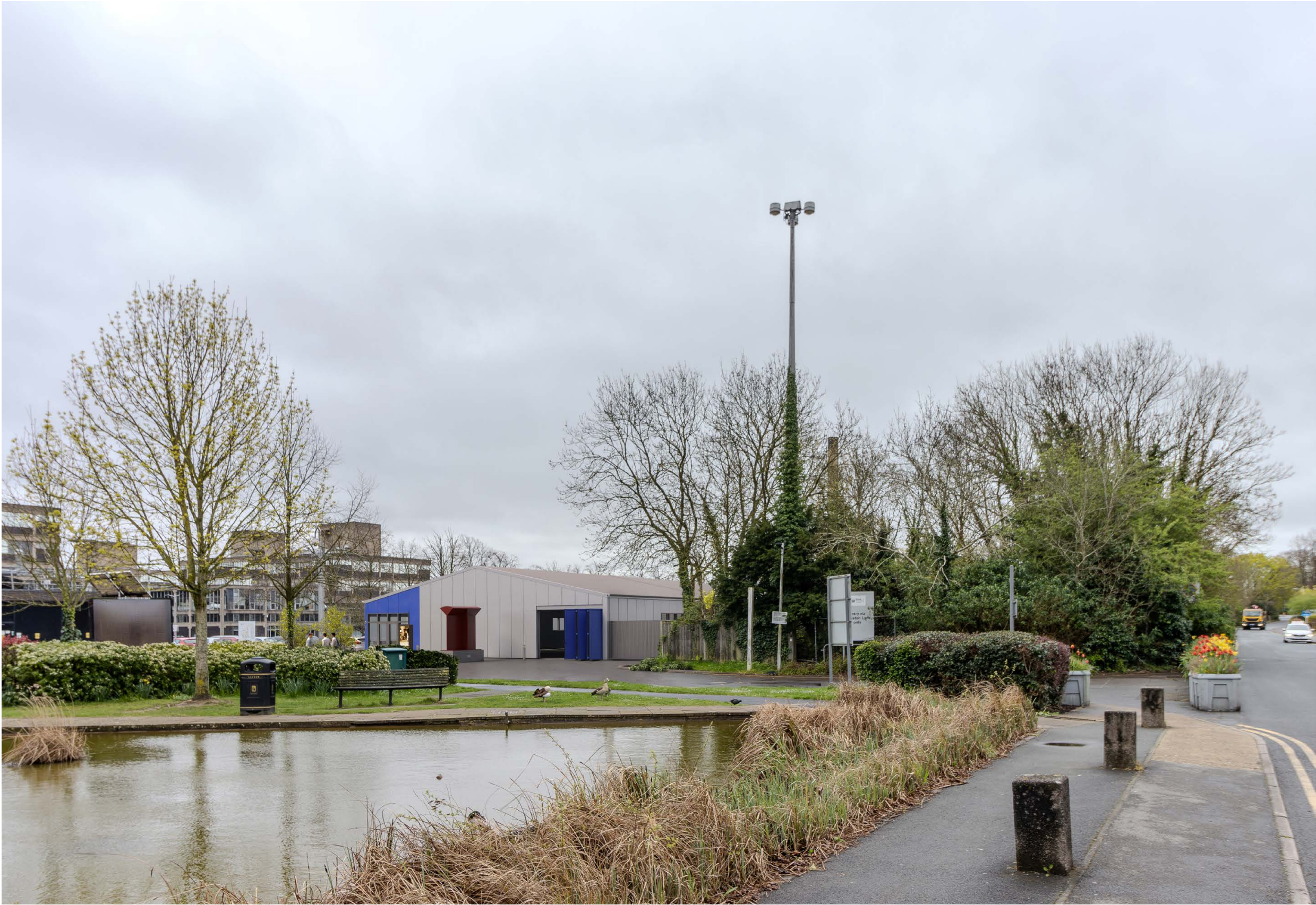
View of south facade of Building 1 from Cleveland Road
