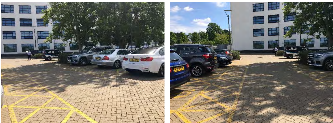
Figure 4.11 – Existing car park with permeable block paving surface (Eastern Gateway)
