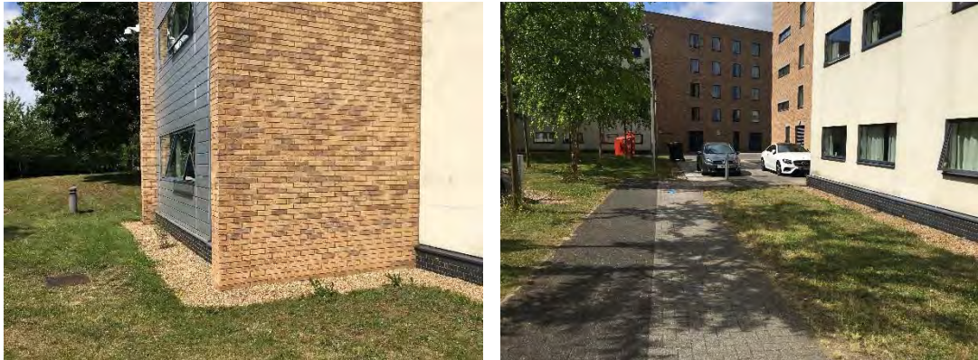
Figure 4.7 – Existing filter drains (Isambard Complex)
