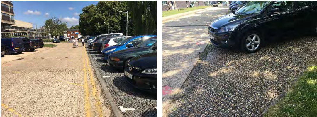
Figure 4.9 – Existing car park with gravel permeable paving grid system (South Loop Road)
