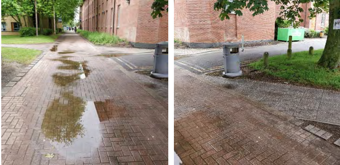
Figure 4.14 –Water ponding on the pedestrian path between the Galbraith Hall and the Gaskell building
