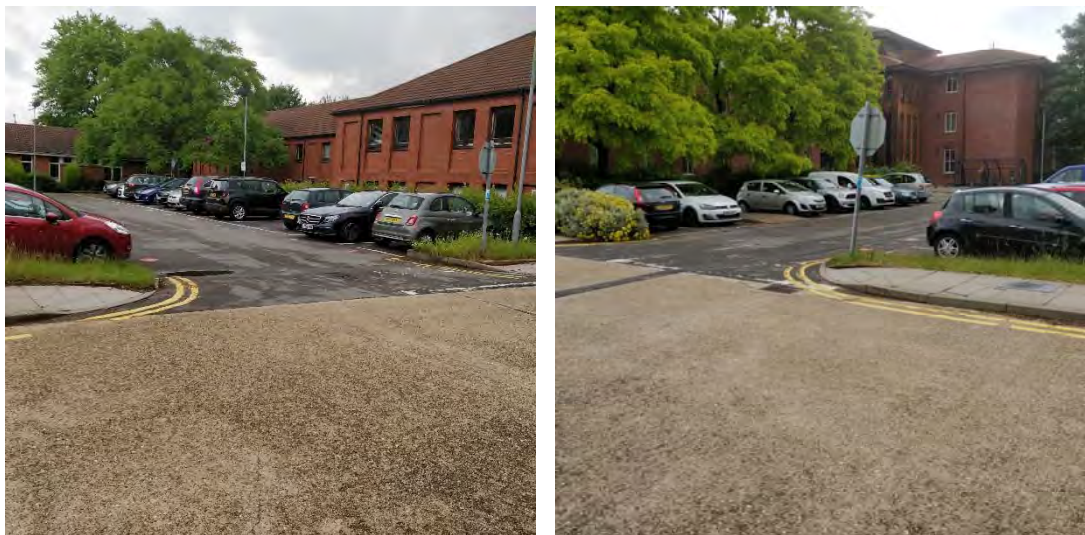
Figure 4.15 – No water ponding after heavy rain at the car park between the Gaskell Building and the Maria Jahoda Building
