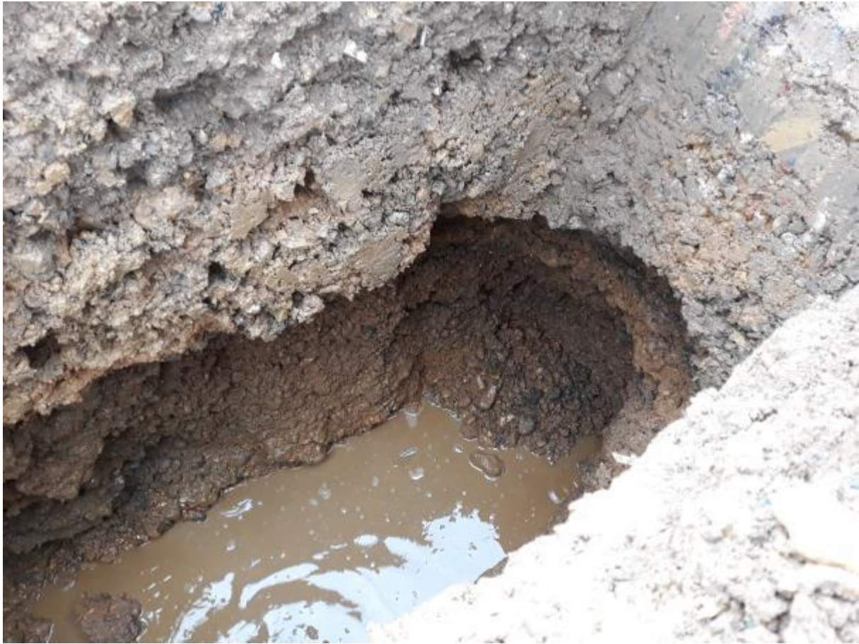
PLATE 14: Groundwater at base of TP204
