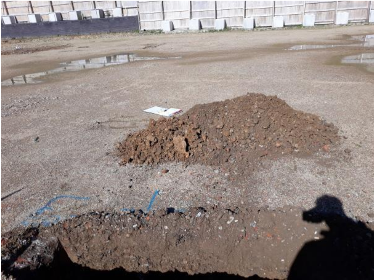
PLATE 7: Stockpile from TP203
