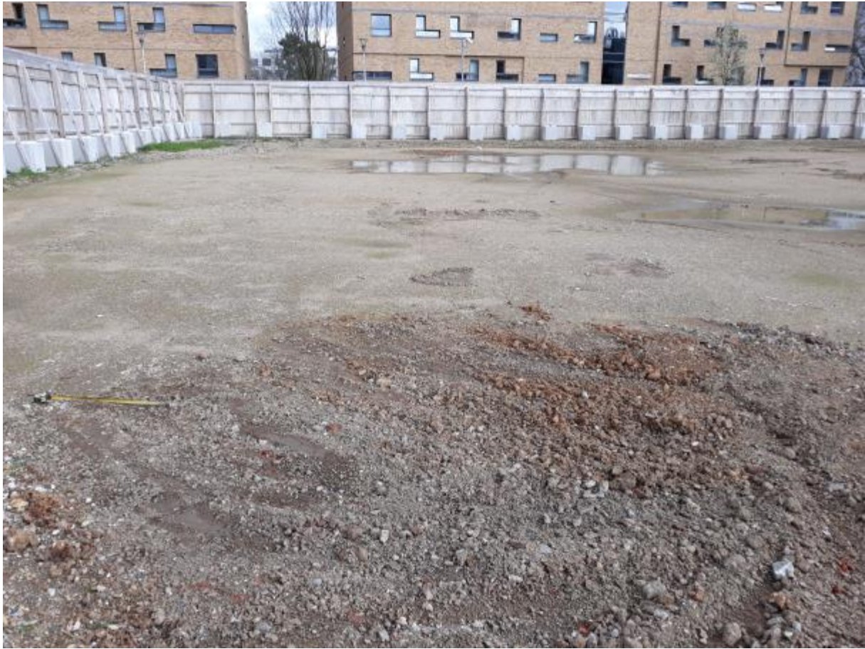
PLATE 15: Overall site view with backfilled trial pit in the foreground.
