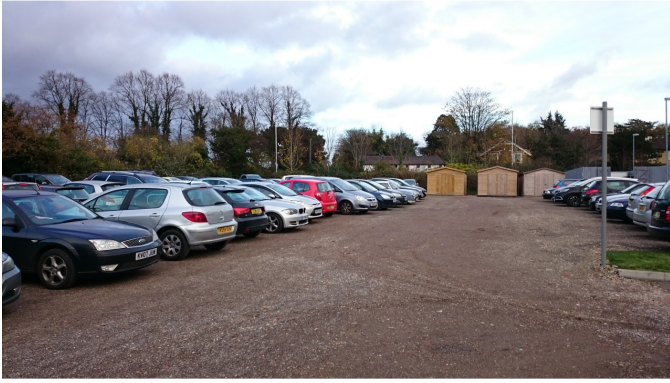
Existing compacted gravel in site I/P10 to be reused
