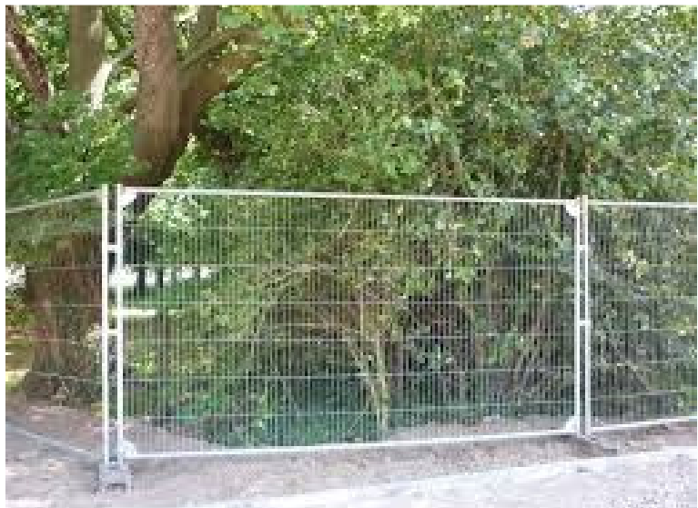
Example of weld mesh panel tree protection
