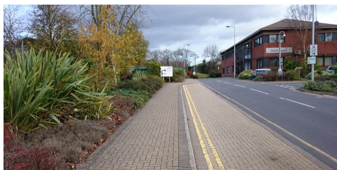
Existing brick paved site in I/P8. Bays to may brickwork pattern.
