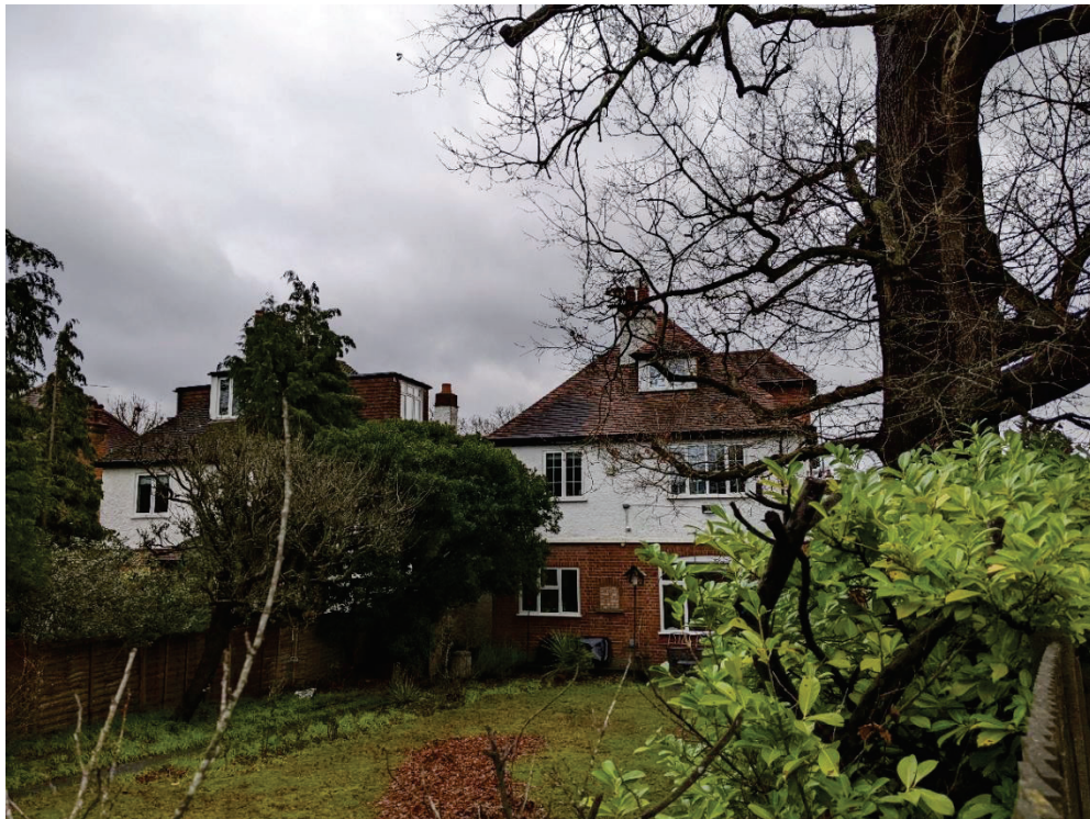
Figure 4: Rear of Application Property as Viewed from Public Footpath
