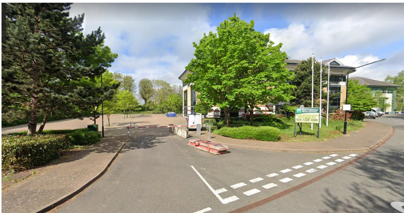
Image 2 – Principal elevation of Waterside House including large car park to the left
