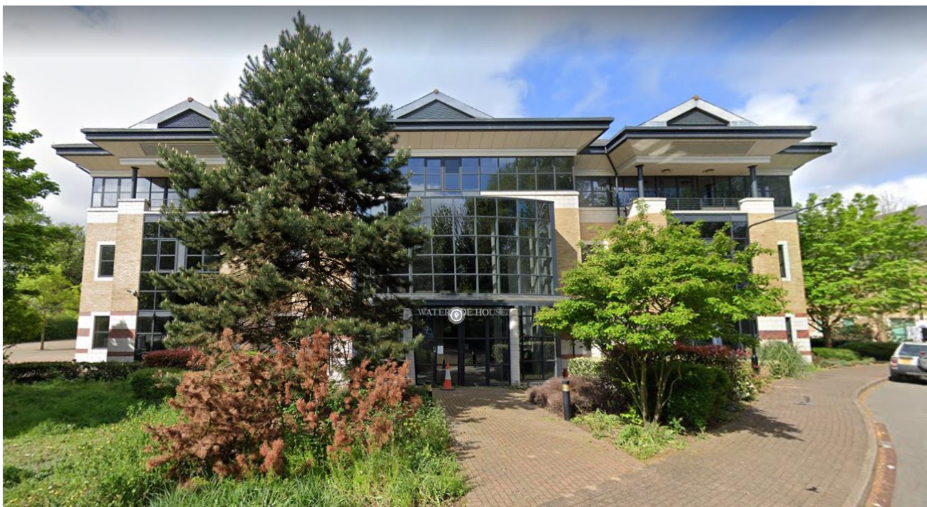
Image 1 – View of front elevation of Waterside House fronting onto Cowley Business Park Road
