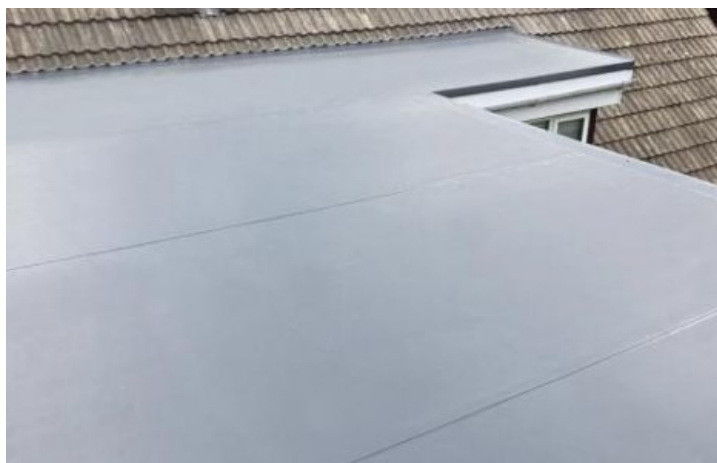
Sarnafil or similar approved single ply membrane with lead colour finish Plots 1 - 3
