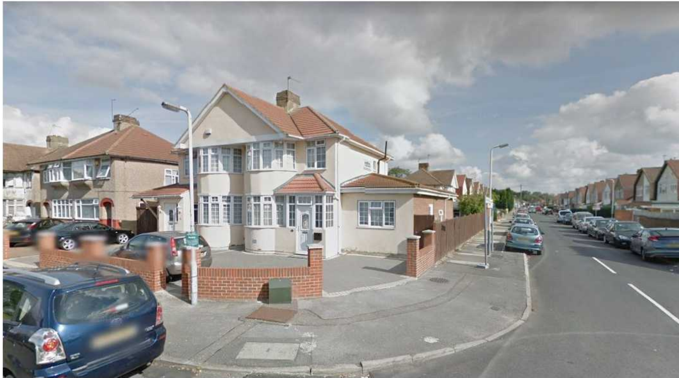
1. View looking east to front of No. 26 Oxford Avenue, showing adjoining properties and existing ground floor side extension.
