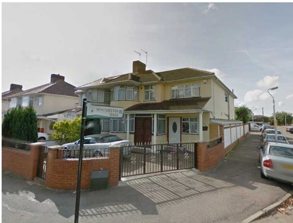
7. View looking south-west to front of No. 23 Oxford Avenue showing double storey side and rear extensions similar to that of the application site.
