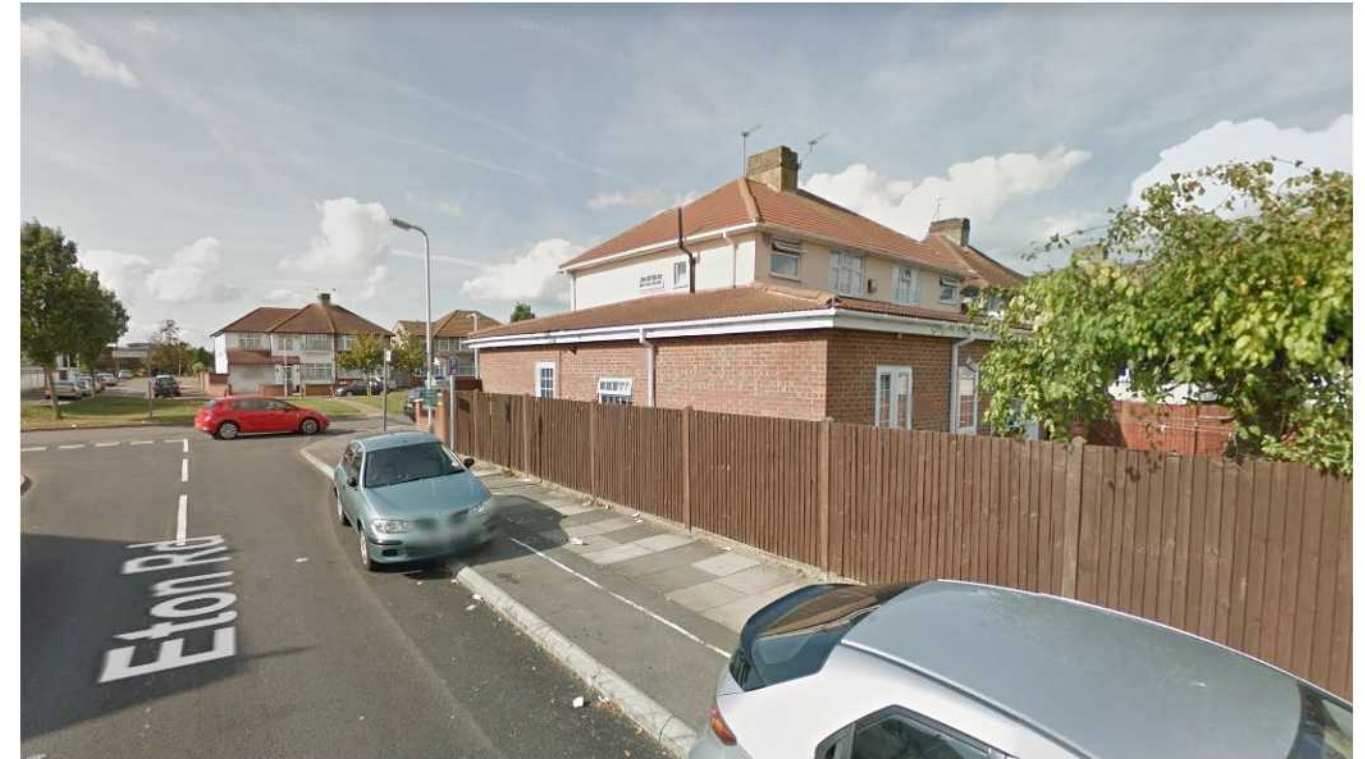
2. View looking north-west to rear of No. 26 Oxford Avenue from Eton Road, showing existing ground floor side & rear extension.
