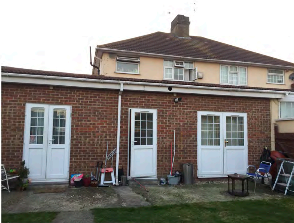
3. View looking west to rear of No. 26 Oxford Avenue, showing existing ground floor rear extension.
