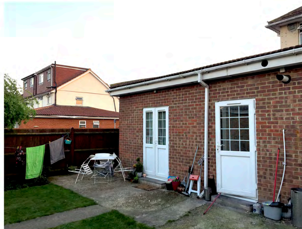
4. View looking south-west to rear of No. 26 Oxford Avenue, showing hip to gable, ground side and rear extensions to No 24 Oxford Ave.
