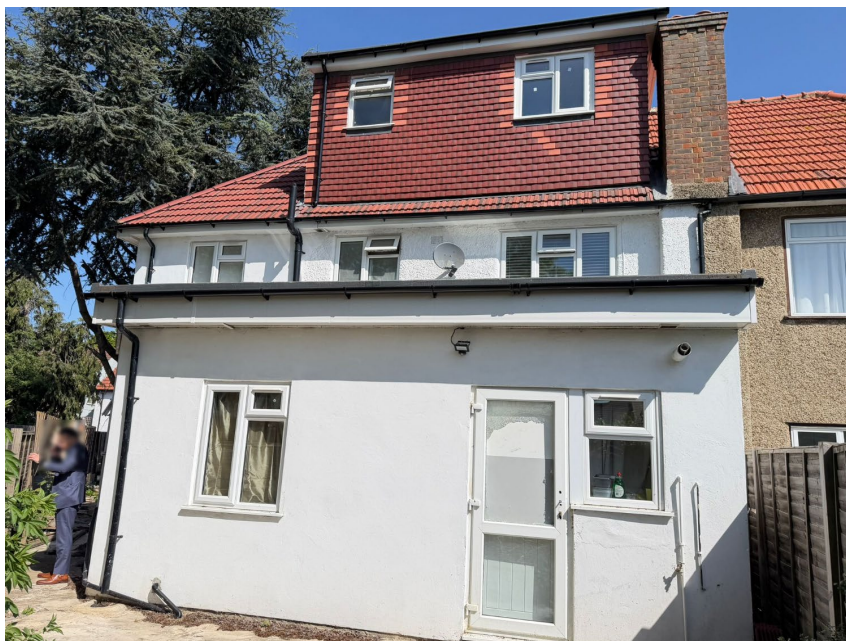
FIG 2: Current photo of the rear of the building
