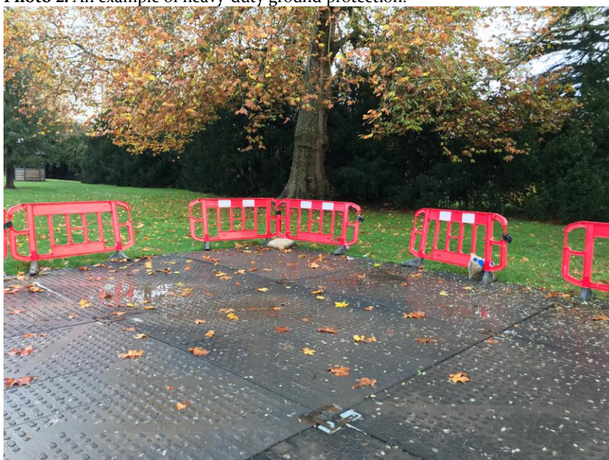
Photo 2. An example of heavy-duty ground protection.
