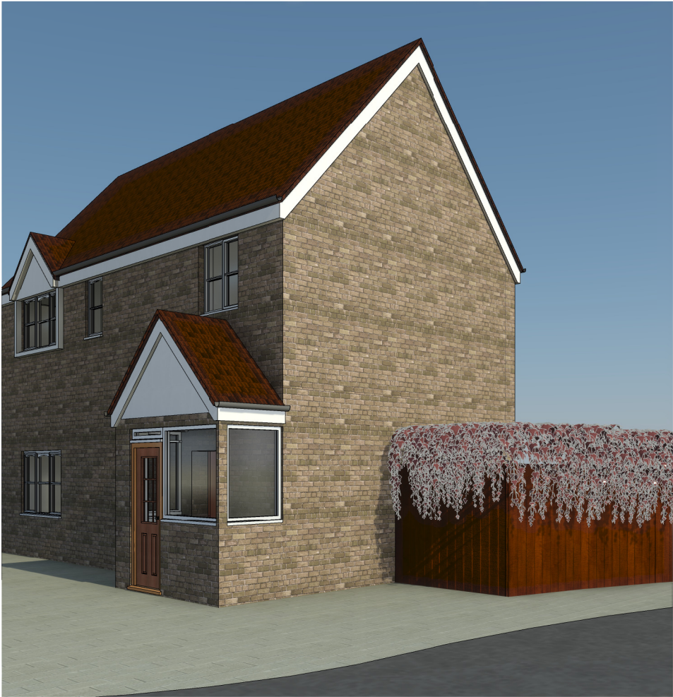
1 BLISWORTH CL - PRE-EXISTING
