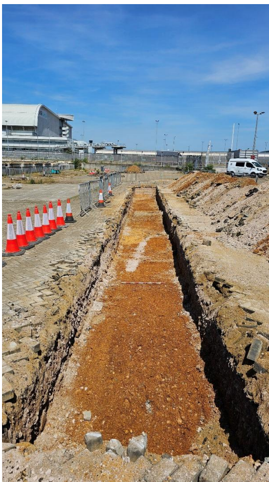
Photo 4 Trench 2, looking north (scale: 1m)
