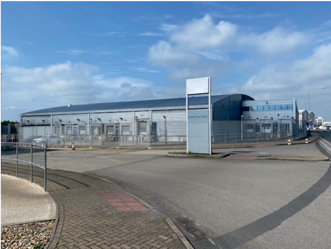
Fig 12 Photograph taken looking south-west, showing the Catering Centre (MOLA photo, 03/06/2021)
