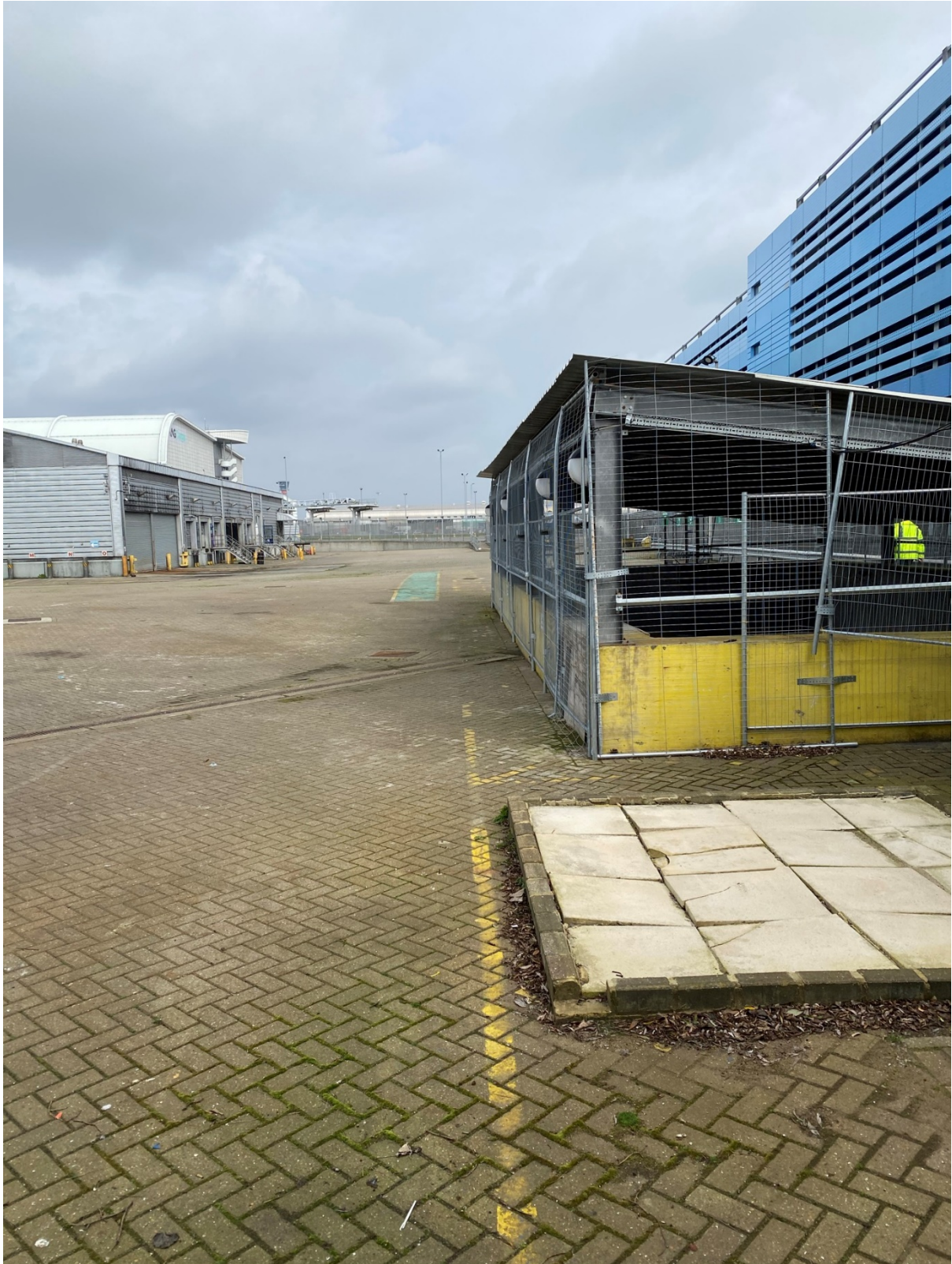
Photo 2 – view from the south east corner of the Site, looking north
