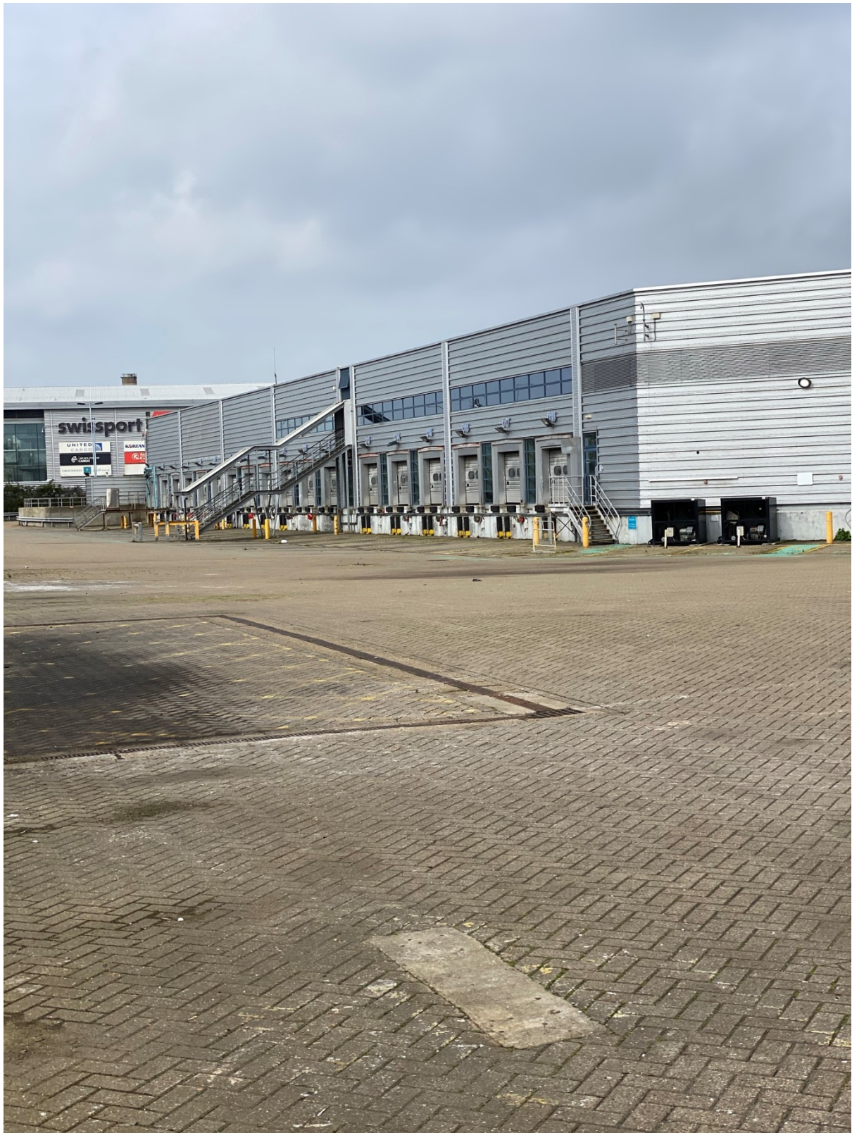
Photo 4 – view from the south east corner of the Site, looking toward the rear of the main building on Site
