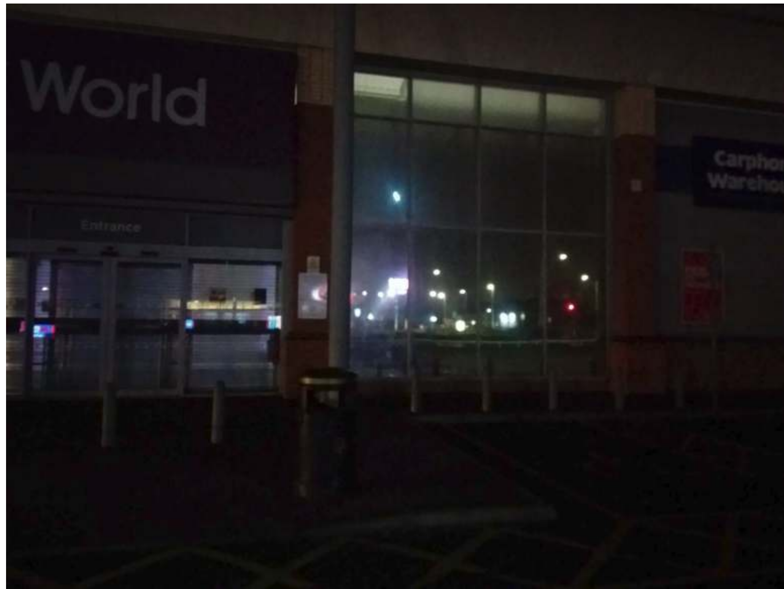
5 FRONT ELEVATION - LHS WINDOWS EXISTING
