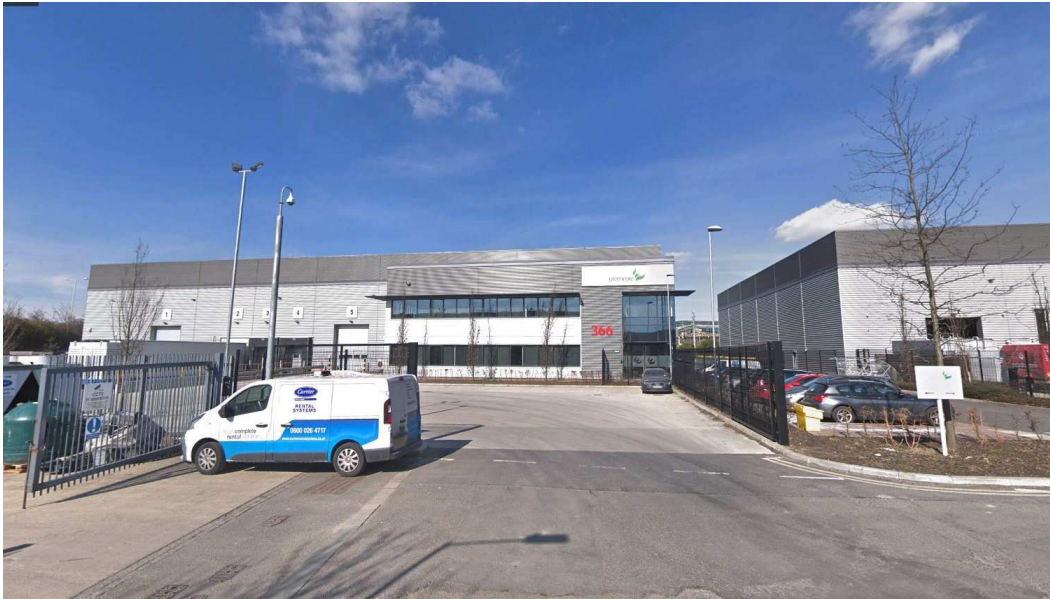
view from entrance gate to service yard
