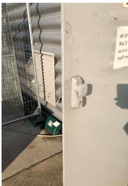
keyed access through fire door
