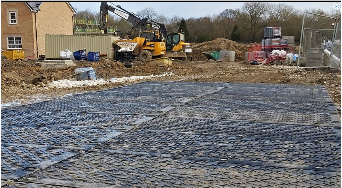
Fig. 3 Ground Guards – Maxi Trak Heavy duty is ideal for the ground protection required here.
