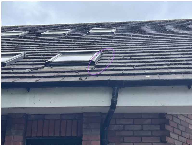
Potential roosting feature: Gaps under roof tiles (Target Note 1).
