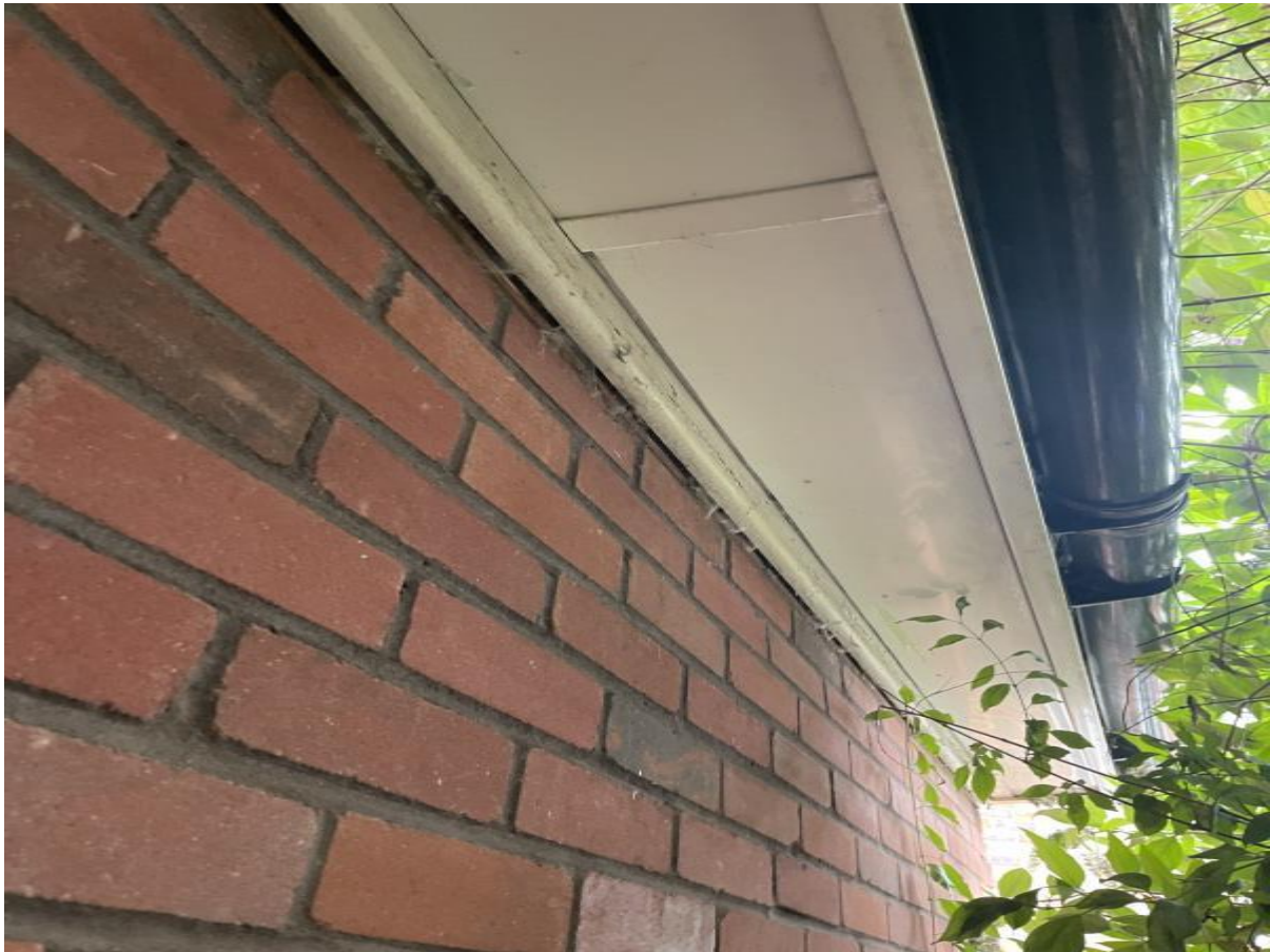
Bat access point: Gaps in fascia and brickwork (Target Note 5).
