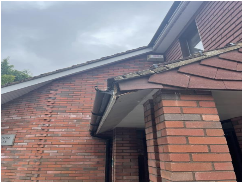
Potential roosting feature: Gap behind soffit box (Target Note 2).
