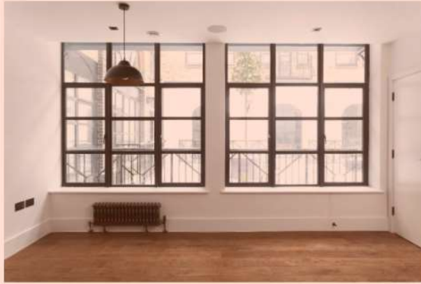
Type:Windows-Smart Architectural Aluminium, Alitherm Heritage Range Grey aluminium window Colour Anthracite Grey RAL7016
