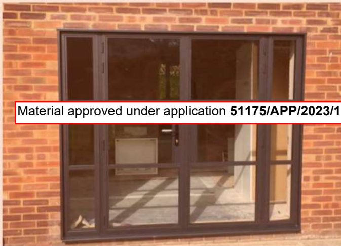
Type:Windows-Smart Architectural Aluminium, Alitherm Heritage Range Grey aluminium window Colour Anthracite Grey RAL7016
