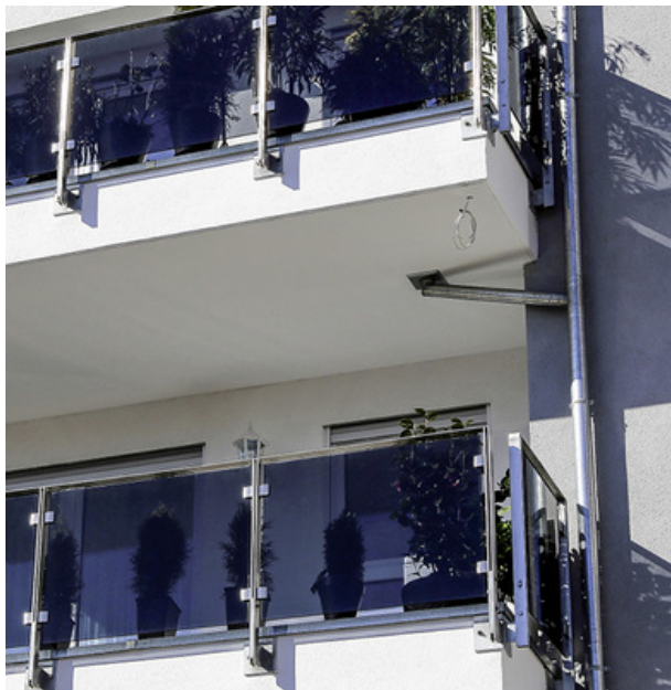
Balcony gutter system from underside of floor. Square guttering, colour RAL7016.
