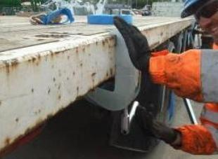
Attach 3 No clamps to the side of the trailer that will be used for loading/unloading, 1 approximately 1m from the headboard, 1 approximately 1m from the rear of the trailer, and the third in the middle of the 2. Then tighten all clamps with handle supplied.
