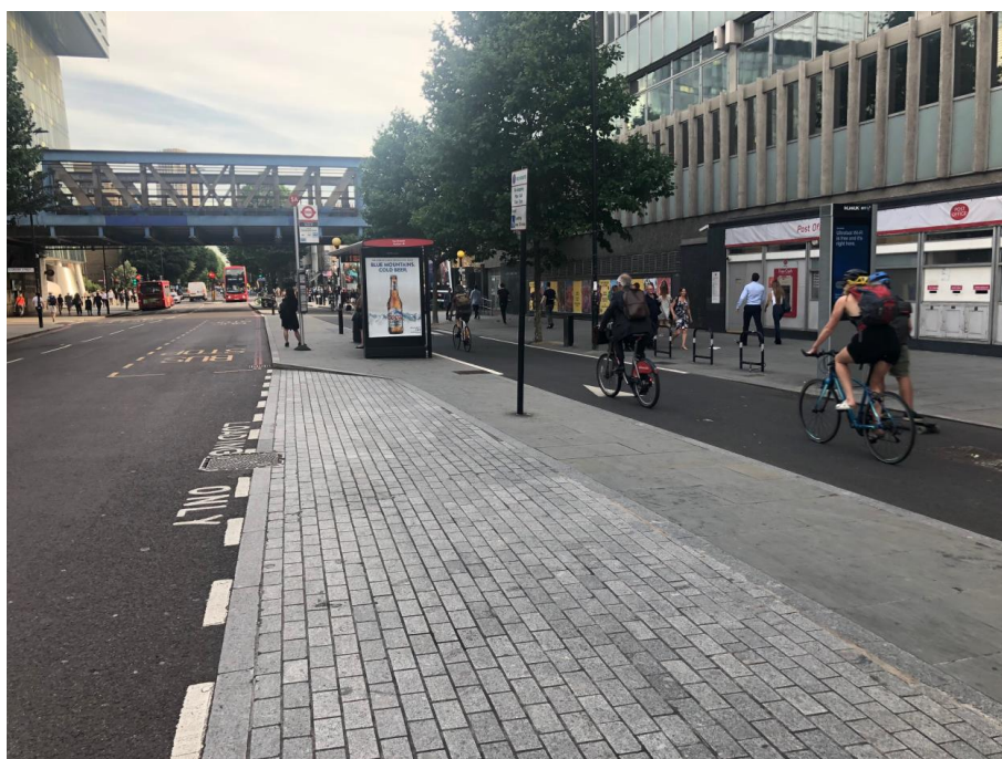
Plate 3.1 – Loading Bay separating Cycle Lane and Carriageway
