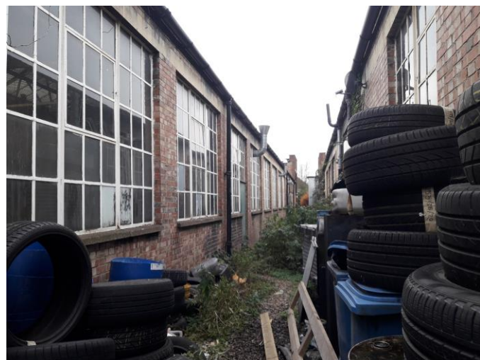
Photograph 3 Western elevation of building and patches of scattered scrub.
