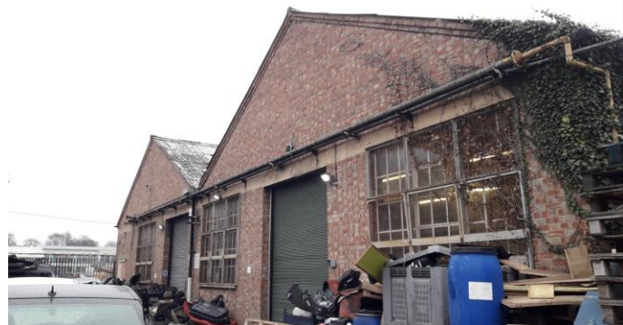
Photograph 2 Northern elevation of building.
