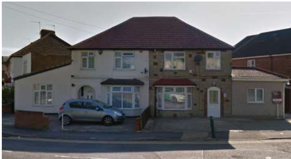
Image 3: Front elevation of 62 Nestle's Avenue and 78 Black Rod Close
