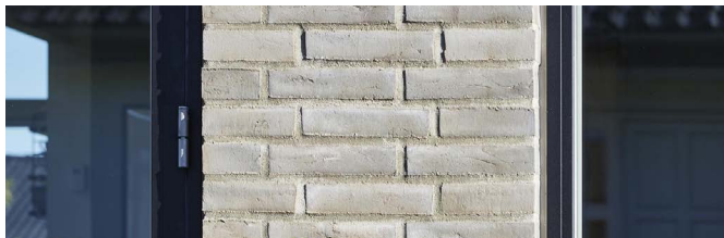
Secondary Material: Inset brick panels in a subtle grey contrast
