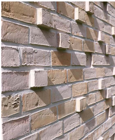
Protruding headers in brick panelling
