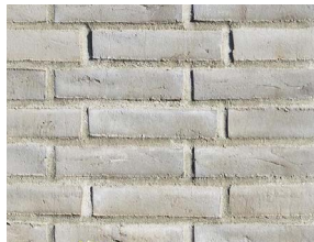
Secondary Material: Inset brick panels in a subtle grey contrast
