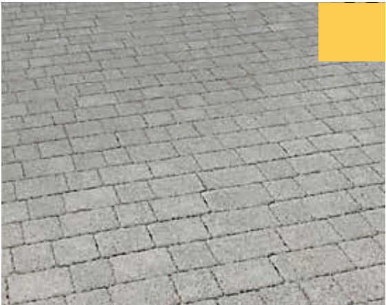
PAVING TYPE 3 : PERMEABLE CONCRETE BLOCK PAVERS
