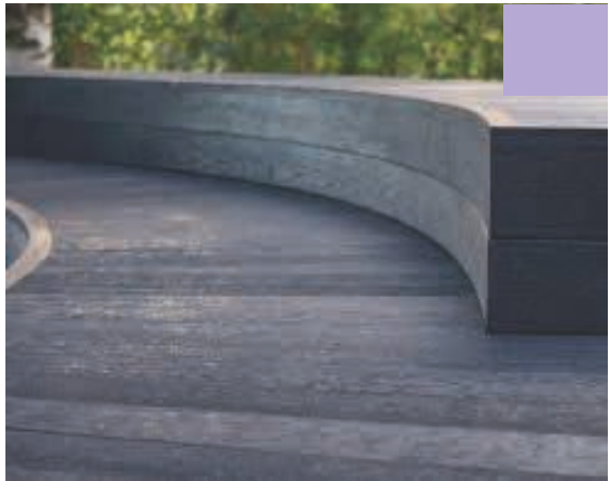
PAVING TYPE 5 : COMPOSITE DECKING
