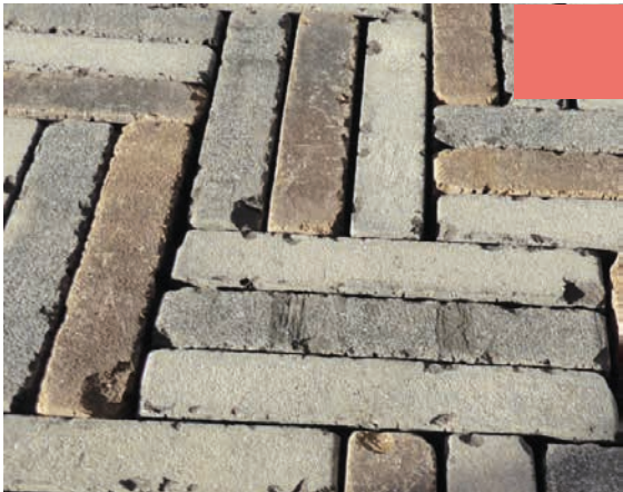
PAVING TYPE 1 : CLAY PAVERS
