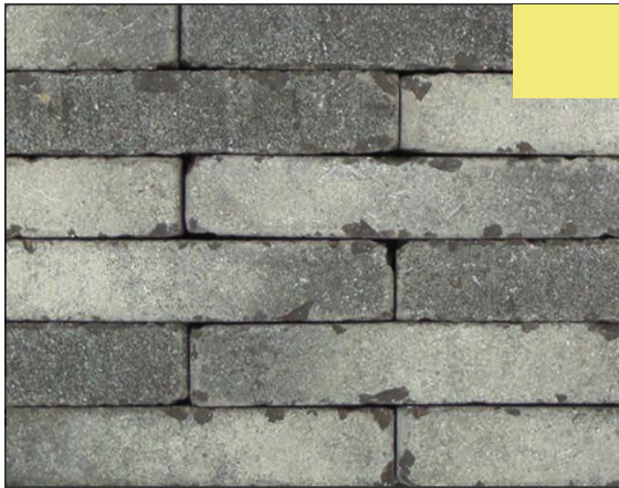
PAVING TYPE 2 : CLAY PAVERS
