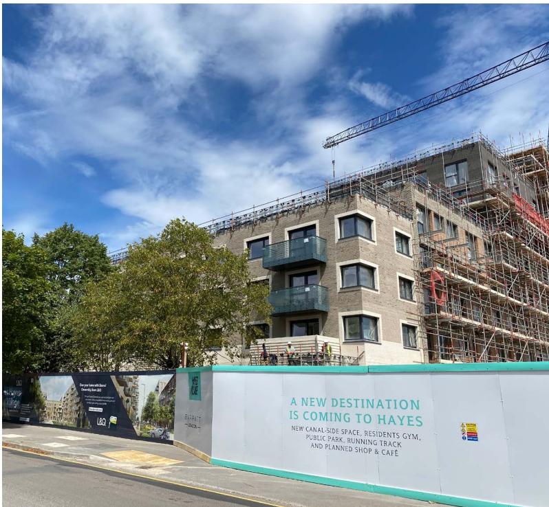
Construction progress on site July 2020
