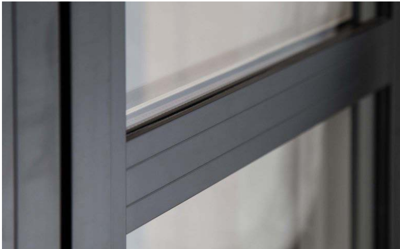
Glazing bars - PPC aluminium glazing bars to the external face and timber styling bars internally
