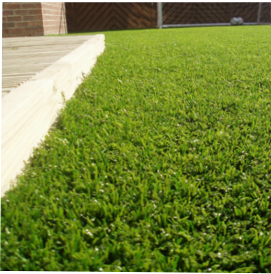
6. Roof gardens- Artificial grass
