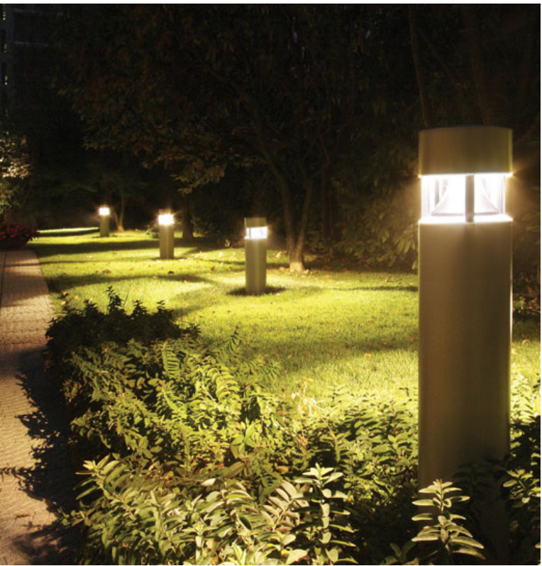
○ Lighting bollards in roof gardens
