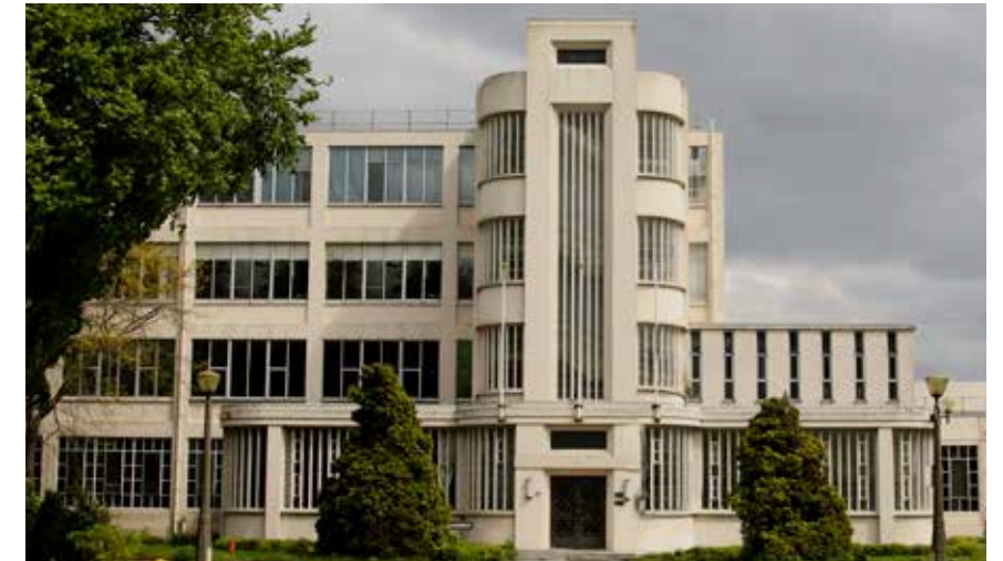
Existing Nestle Factory Building
