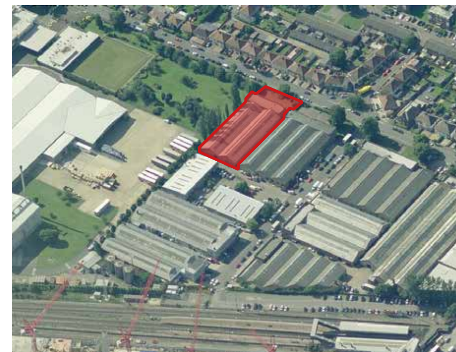
Aerial View from the North
