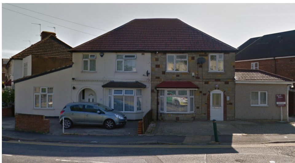
Image 3: Front elevation of 62 Nestle's Avenue and 78 Black Cod Road
