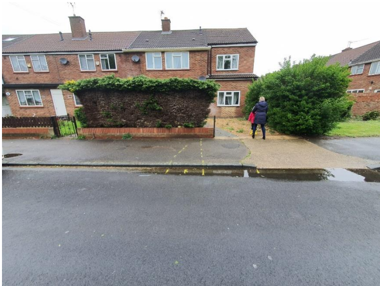
Photograph 01 – Front of the house
