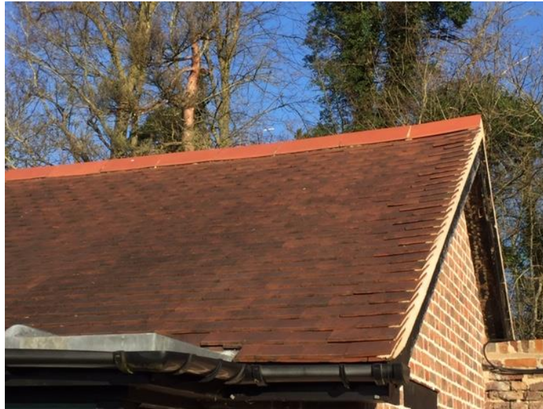
Redland Rosemary roof tiles with terracotta ridge.
