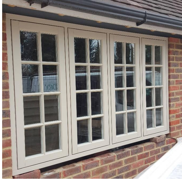
Stained hardwood window frames.
