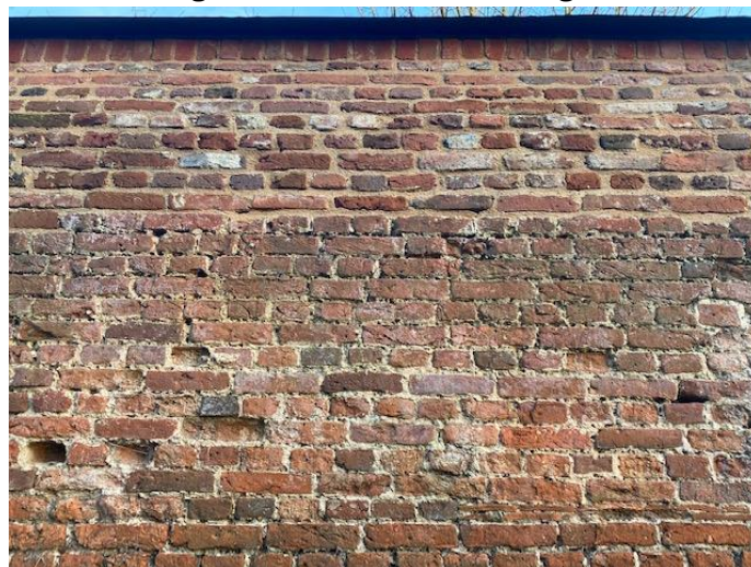
Existing and new reclaimed Facing bricks.
