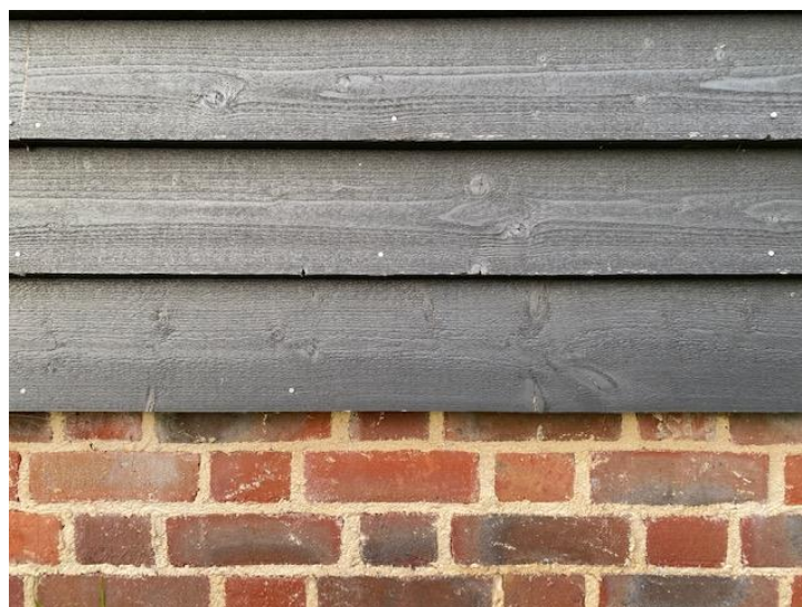
Ibstock Hamsey facing brick and timber cladding to outbuilding
